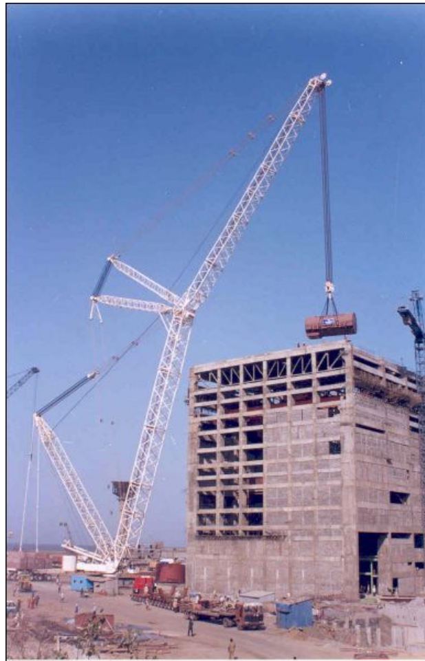
Erection of Turbo Generator
