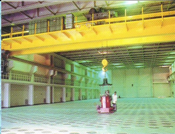
Solid Storage Surveillance Facility
