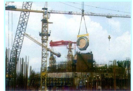
End Shield Erection
