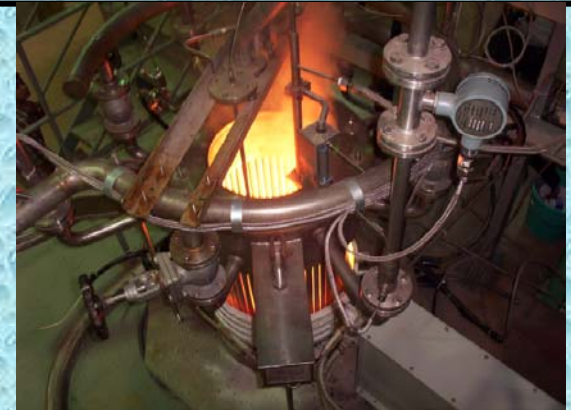
Cold Crucible Induction Melter : Engineering demonstration facility
