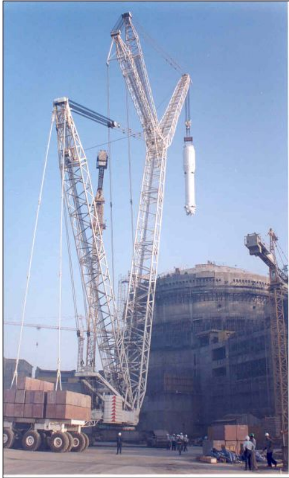
Steam Generator Erection
